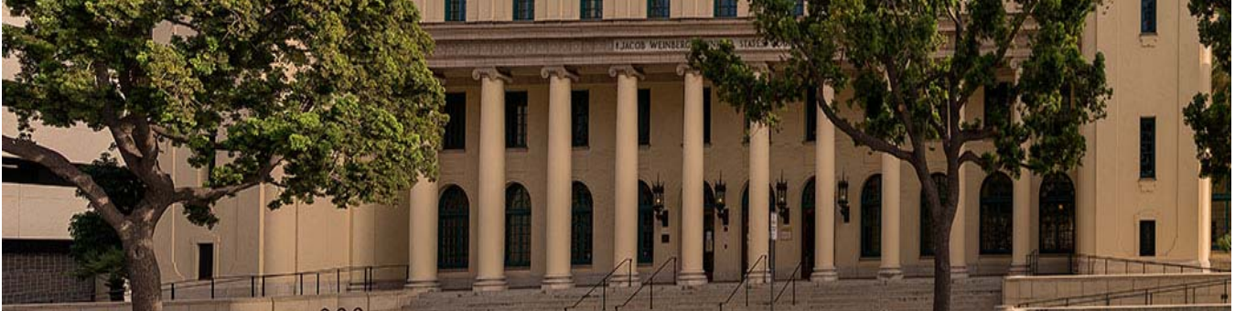
The old Federal Building and United States Courthouse now named the Jacob Weinberger United States Courthouse
