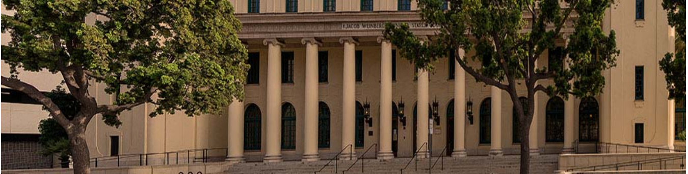
The old Federal Building and United States Courthouse now named the Jacob Weinberger United States Courthouse
